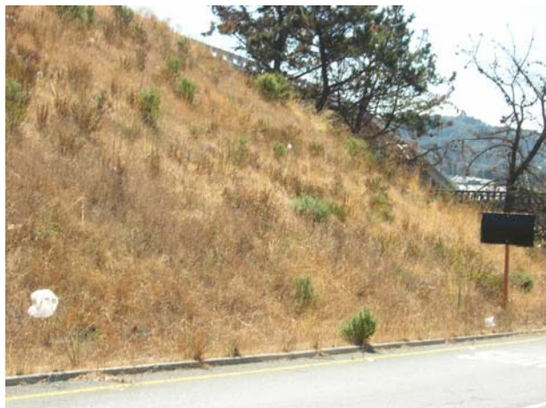
Figure 5B, Fully vegetated 1.5:1 Slope – Erosion Control (Type B)
