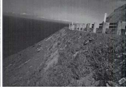
Figure 3B. Natural colonization of adjacent vegetation. 1:1.5 (H:V) Slope face gradient. 04-Son-01 May 1998
