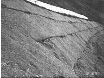
Figure 3. Completed 1:1.5 Wrapback constructed slope
