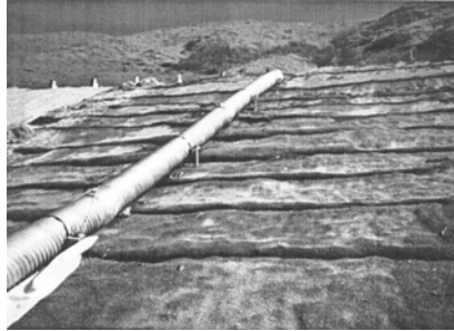
Figure 3A. Wrapback slope with drainage down drain
