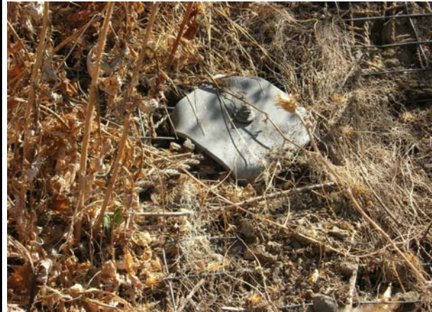
Figure 5A, Anchor plate over wire mesh
