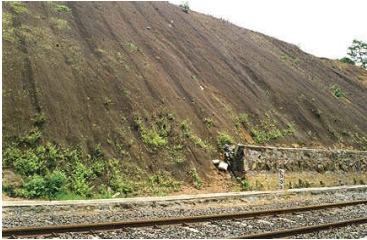
Geotextiles laid site- Konkan Railway
